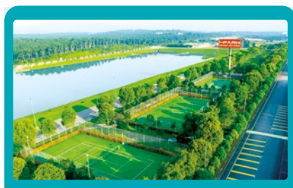
i-Park @ Senai Airport City
