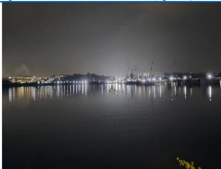
Figure 22: RTS Link across the Straits of Johor (night view)
