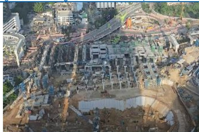
Figure 36: Bukit Chagar station RTS Link site (June 2024)
