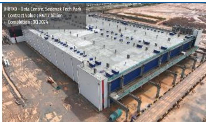
Figure 41: Project site of JHB1X0 data centre in STeP in Feb 2024
