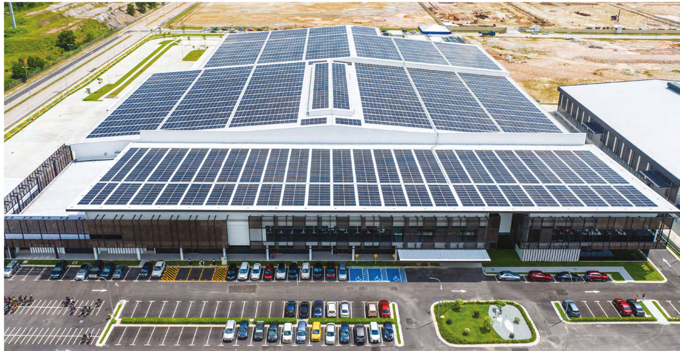
A medical devices facility spanning over 12 acres in i-TechValley
