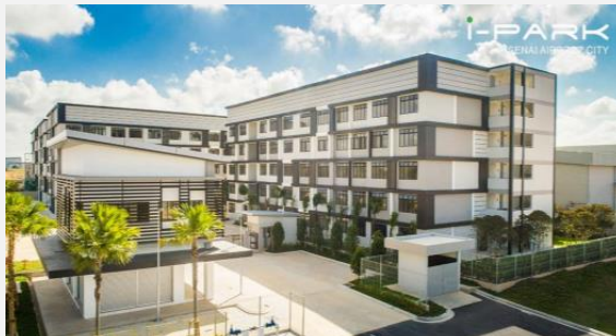
i-Park@Senai Airport City
