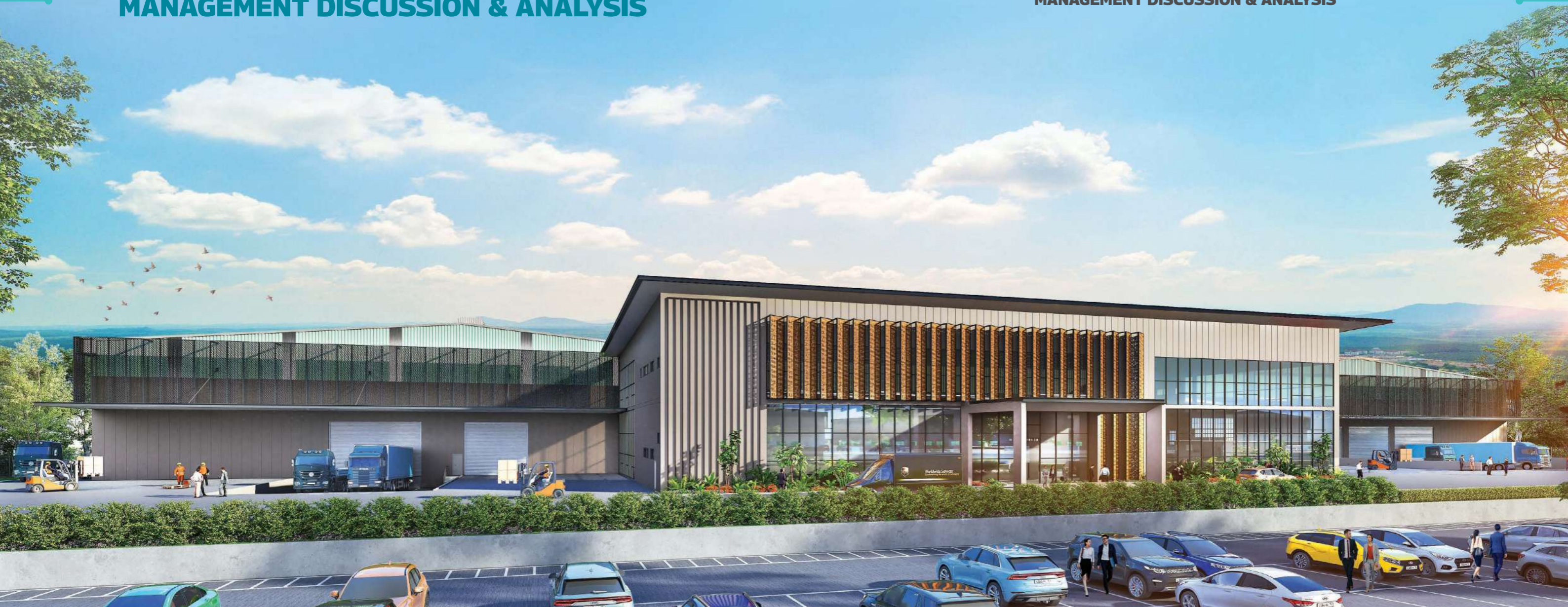
i-Park@Senai Airport City (Phase 3) – 10-acre-and-above factory
