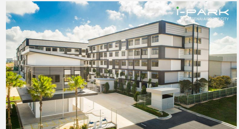
i-Park@Senai Airport City
