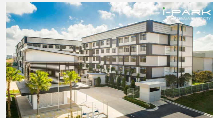
i-Park@Senai Airport City
