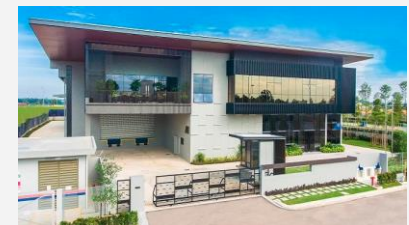
i-Park@Senai Airport City
