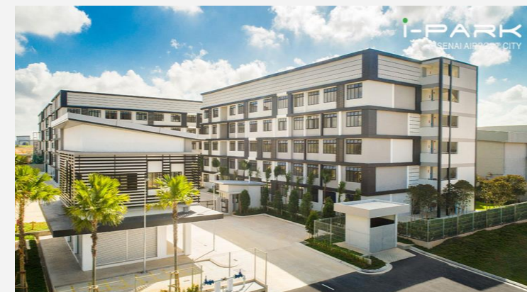
i-Park@Senai Airport City
