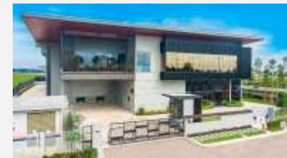
i-Park@Senai Airport City
