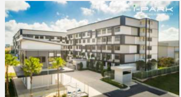
i-Park@Senai Airport City
